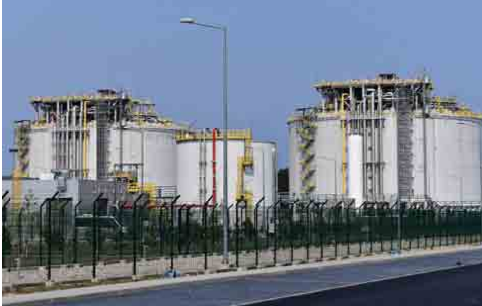
PRESIDENT LECH KACZYŃSKI'S LNG TERMINAL IN ŚWINOUJŚCIE, POLAND, APRIL 24, 2019.
